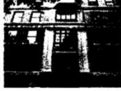
Jackson Shore East Facade Center Bay
